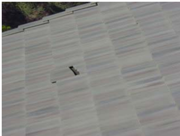
Picture 3: Example of broken tiles.
